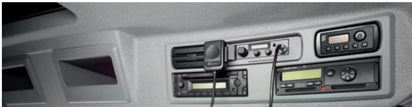
Communications HQ – the standardised DIN slots house the digital tachograph and radio. This is also where the CB two-way radio that is available ex factory and FleetBoard® – the vehicle, fleet and transport management system from Mercedes-Benz – can be installed
